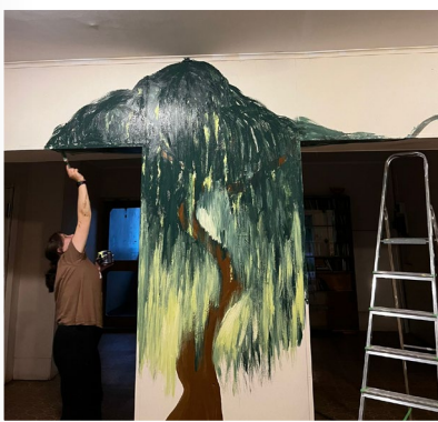
Renovating the hall ©Rita Eglite
