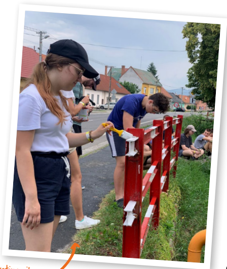
Renovating village ©Denis Válek
